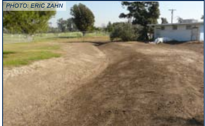
Figure 4. Bioswale Before Planting
