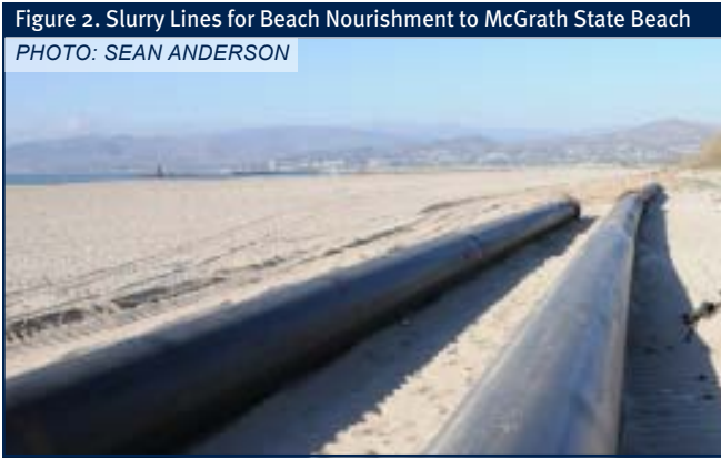
Figure 2. Slurry Lines for Beach Nourishment to McGrath State Beach
