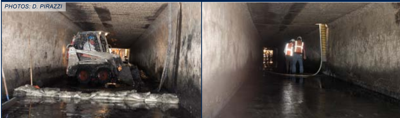
Figure 7. 1,000-Foot Culvert: During and Post-Cleaning
