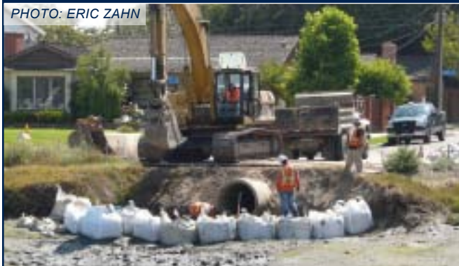
Figure 5. 4th Street Storm Drain Improvements
