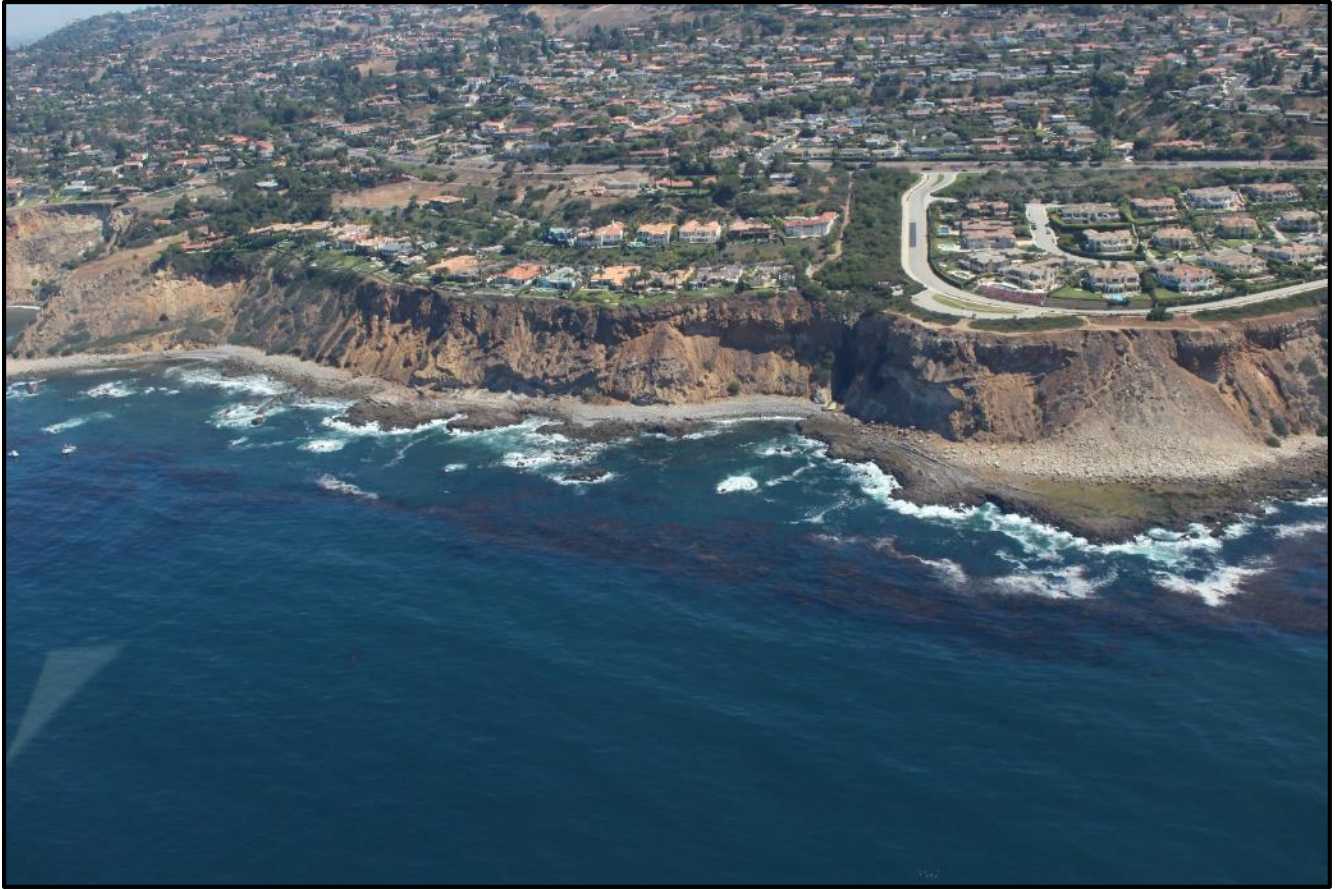
Figure 73 (Site: Marguerite, Date: 04/28/2015, Restoration In Progress, GPS: 33.757, -118.418)
