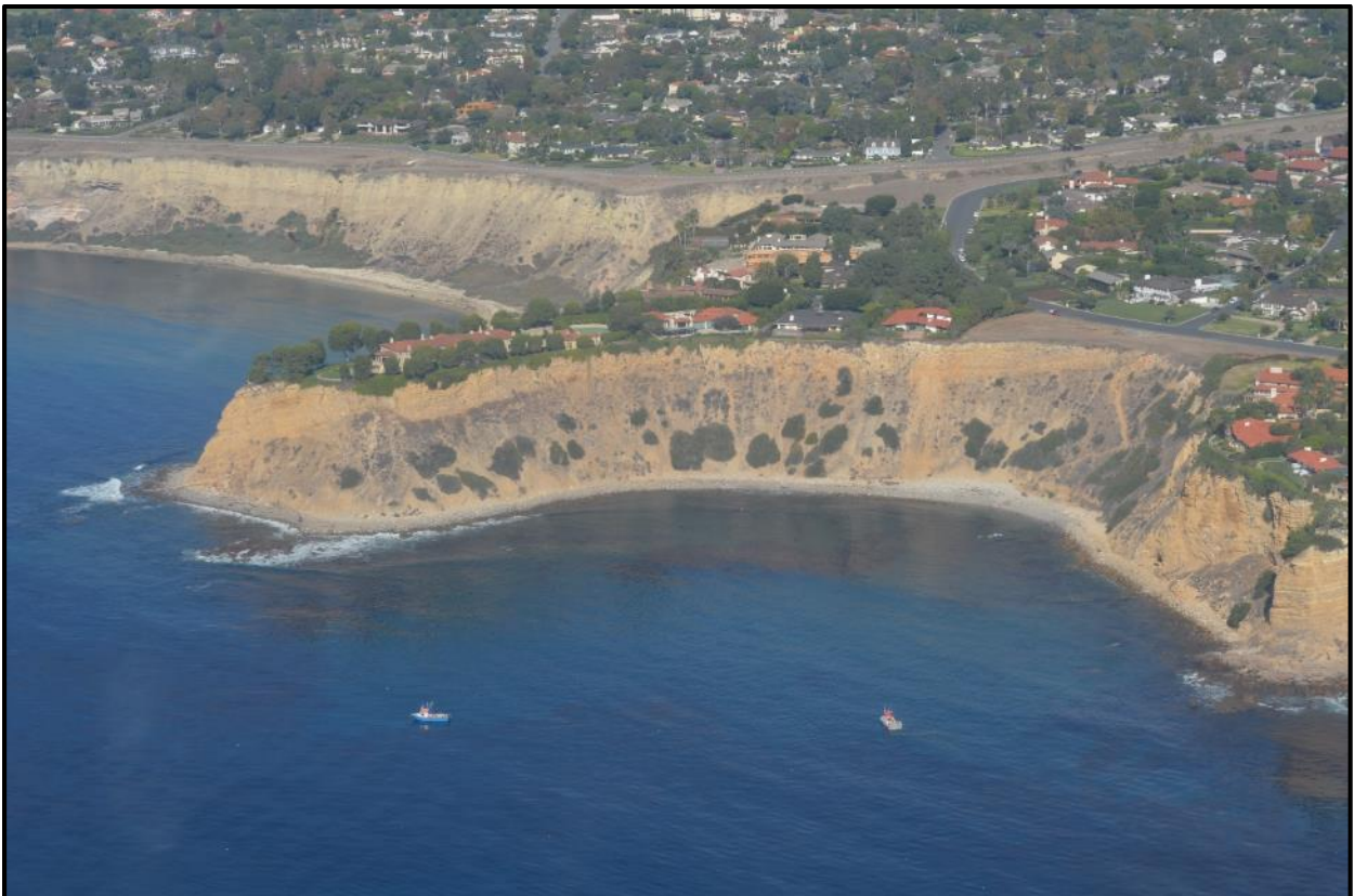
Figure 68 (Site: Honeymoon Cove, Date: 11/07/2013, Pre Restoration, GPS: 33.794, -118.376)
