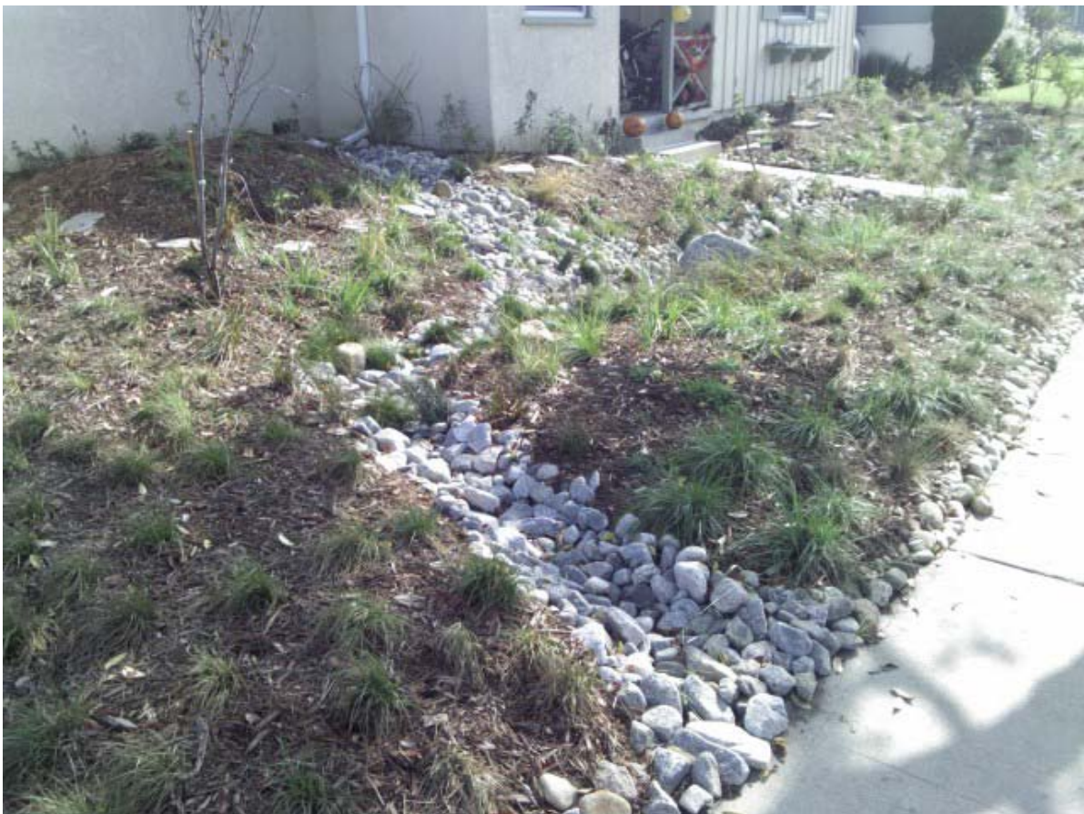
Figure 2.9 Completed rain garden at Culver City residence.
