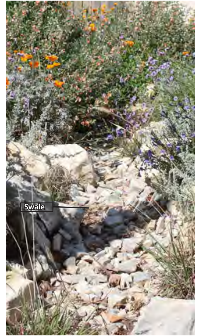
A swale directs water from the downspout to the rain garden. Many swales use rocks that create a dry creek bed look.
