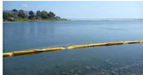
Turbidity curtain worked as designed Checked daily by CDPD and SMBRC staff
