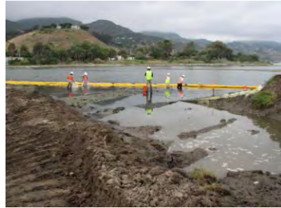
Seined between turbidity curtain and dike installation "A" to "B" channels
