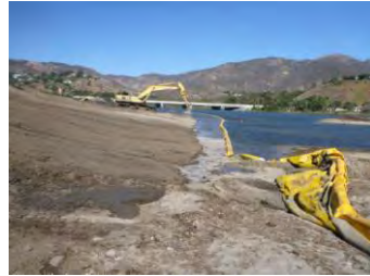
Turbidity curtain worked well during bank contouring
