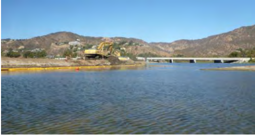
Excavators filled trucks to move fill
