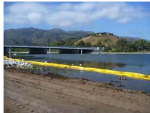
Turbidity Curtain deployed end of day 14 June 2012
