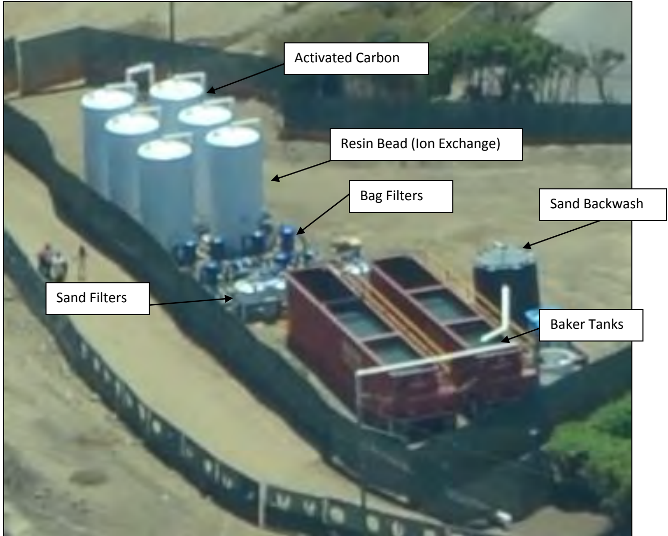
Figure 20. Aerial photo depicting water treatment plant.
