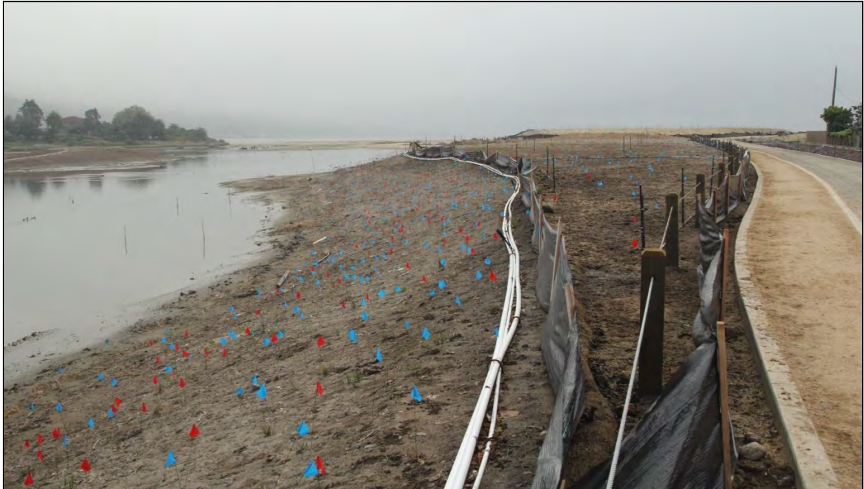
Figure 54. Photograph of Photo Point 2, bearing 75° on 15 March, 2013.
