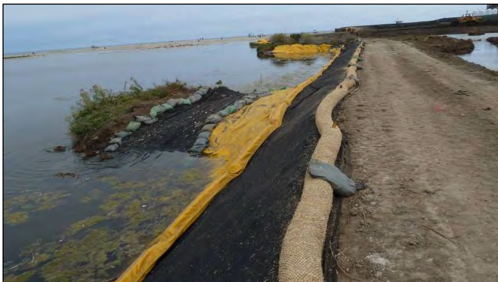
Figure 26. Photo of turbidity curtain while the main Lagoon was tidally influenced (open berm condition).
