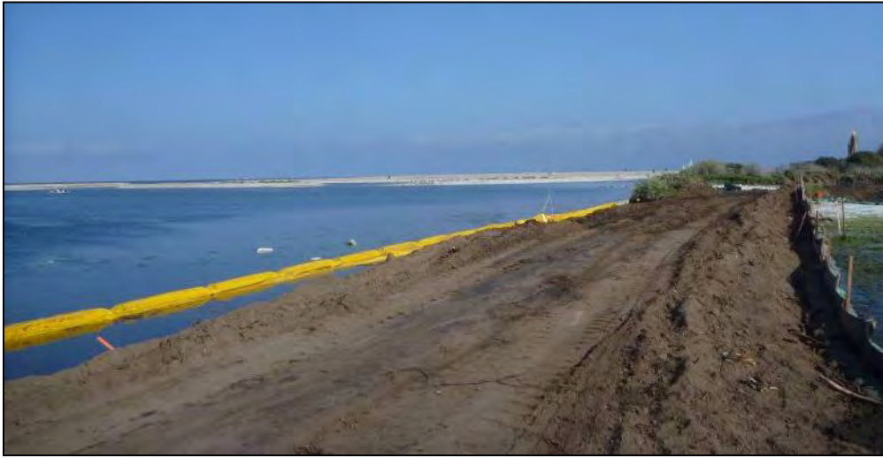
Figure 25. Initial deployment of the turbidity curtain on 14 June 2012.
