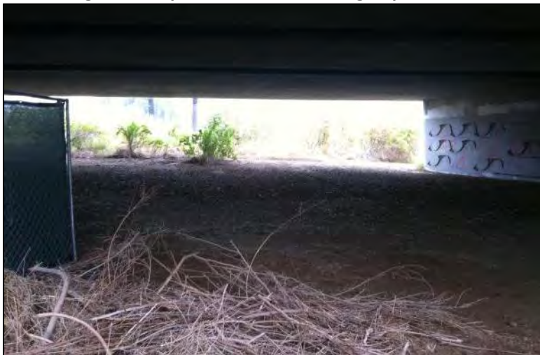
Gates were installed at the NE corner of the project site 6/12/11 to allow wildlife to relocate out and upstream of the construction area (6/13/12).
