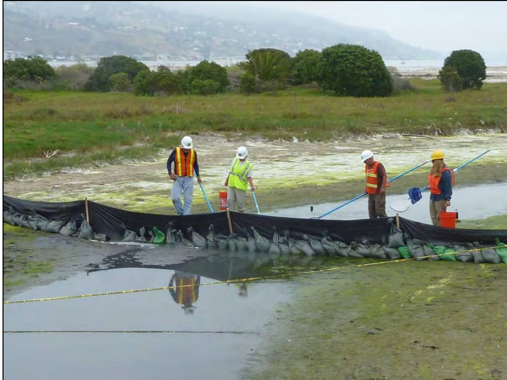
Figure 24. Photo of fish exclusion fence and sandbags.
