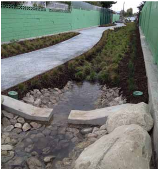
FIGURE 7: Elmer Avenue Paseo on December 12, 2012. PHOTO: NANCY L. C. STEELE
