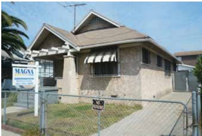
FIG. 1A. The original 100-year-old house before the transformation.
