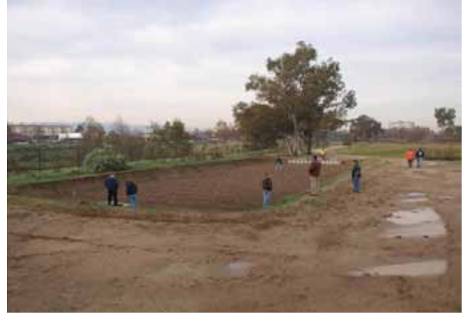
FIG. 7. Post construction of the Modular Wetland System site.
