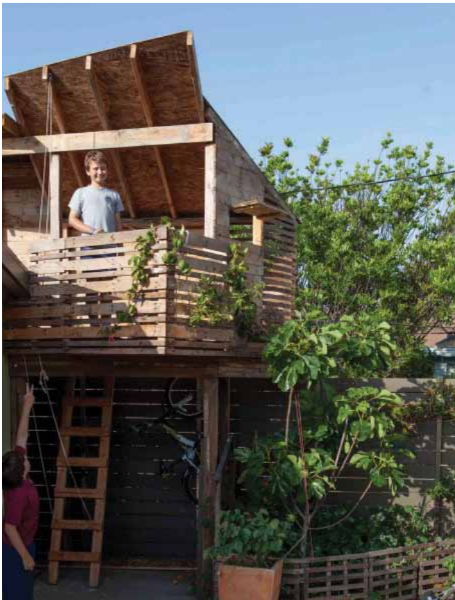
FIG. 17. A tree house made with recycled wood lath and pallettes, next to a young fig tree and the berry patch.
