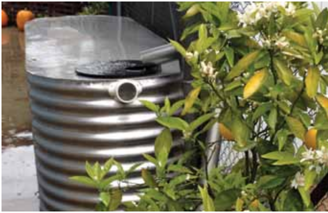
FIG. 9. A 500 gal. stainless steel cistern and overflow diverter positioned in a prominent location on the site to encourage discussion.
