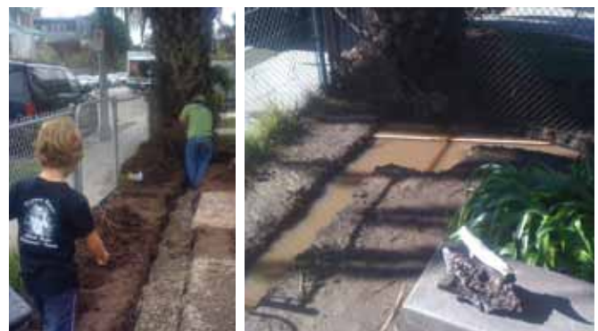
FIG. 6A. Percolation trench during construction showing filter fabric and gravel.
