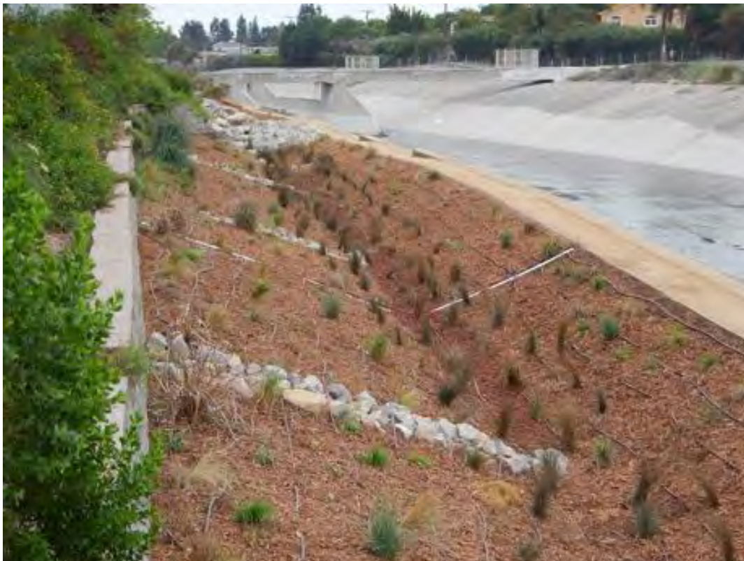
Figure 1.2.1-3. The newly planted Culver City rain garden located along the Ballona Creek. This 1000-ft rain garden intercepts runoff from commercial buildings and parking lots located along Jefferson Blvd. Photo: Ivan Medel, The Bay Foundation
