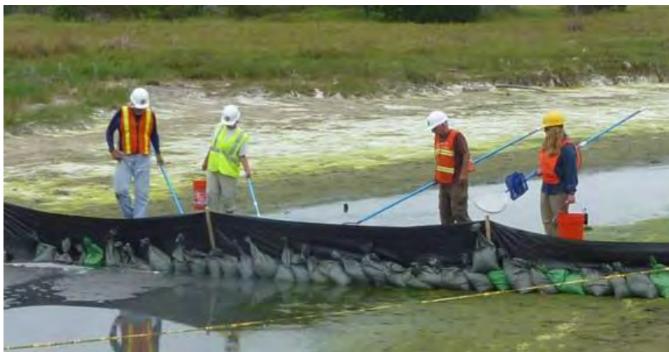
Figure 2.2.2-2. Project staff removing any fish trapped behind an exclusion barrier prior to pumping water from the channel. Photo: Abramson et al. 2013.
