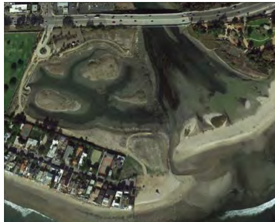
B. Post-Project, December 10, 2013
