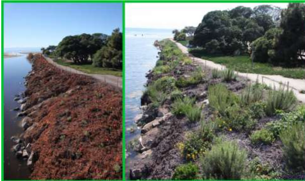
Project site (looking south) after removal of plastic sheeting and initial installation of native plants.
