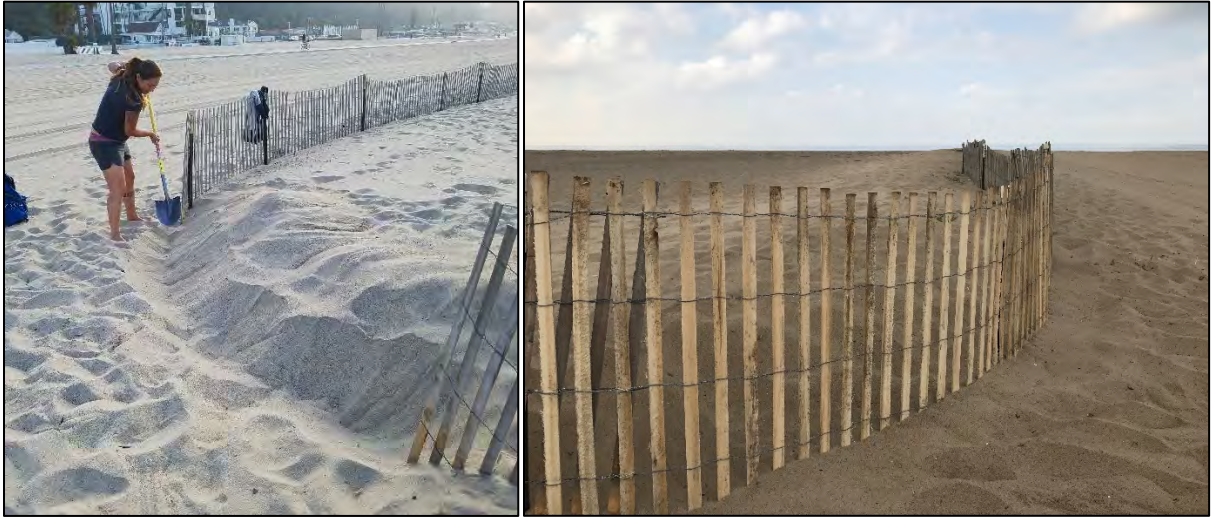
Figure 51. Fence repair before (left) and after (right) on 3 October 2017.
