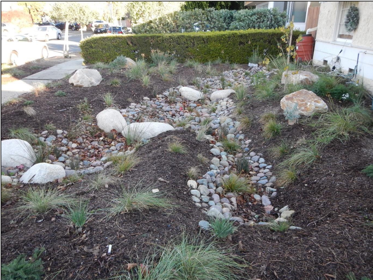
Figure 44. Residential rain garden installed and monitored as part of the MWD grant funded project.
