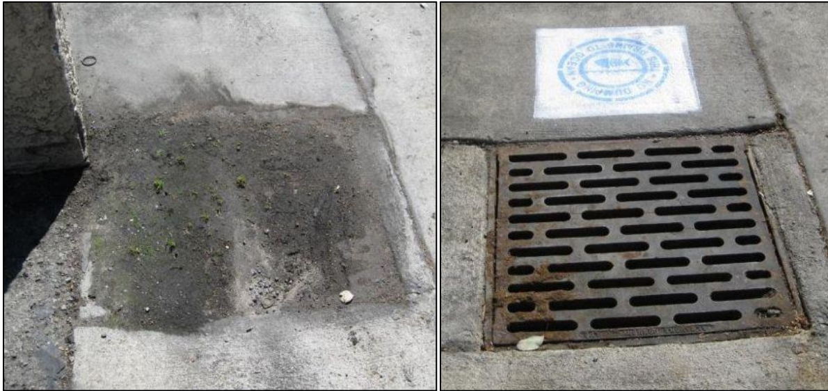
Figure 36. Before and after installation of a storm drain.
