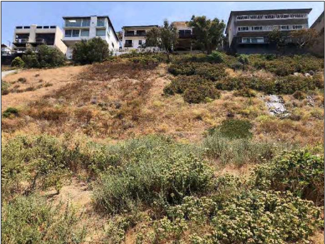
Figure 7. Photo taken of hillside during Year 6, approximately one and a half years after revegetation activities (3 June 2022).
