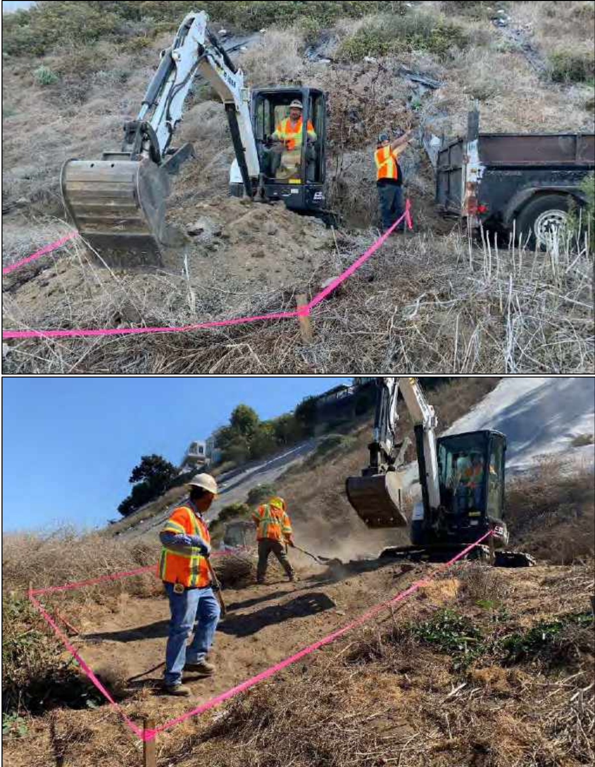
Figure 36. Photographs of the sediment and trash piles immediately before (top) and after (bottom) after removal from the restoration site (13 October 2020).
