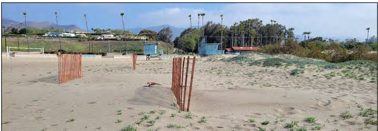
Figure 11. Sand fence segments installed at Zuma Beach (30 March 2021).
