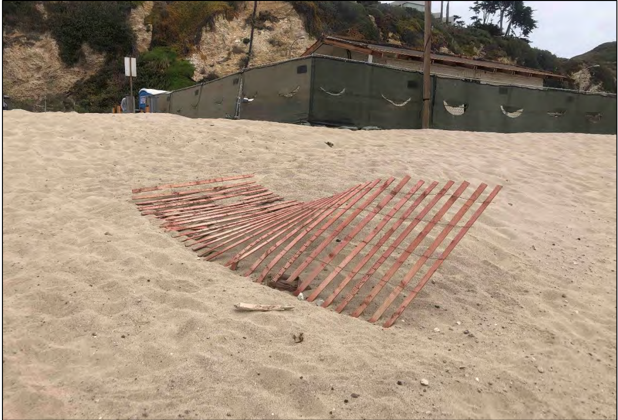
Figure 57. Fallen sand fence (26 April 2021).
