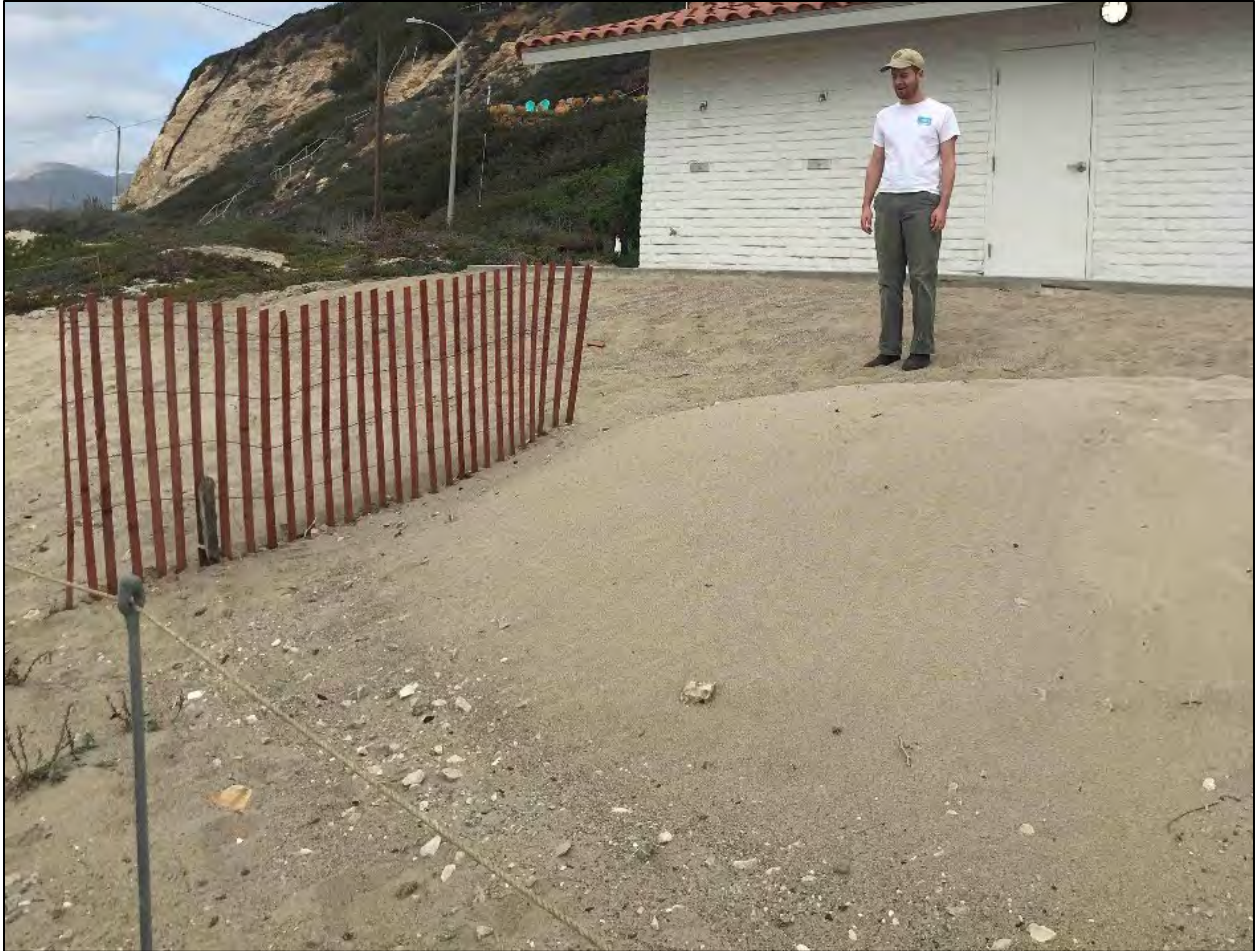
Figure 12b. Photo of sand accretion from sand fencing installed at Point Dume Beach approximately 9 months after implementation on 9 November 2021.
