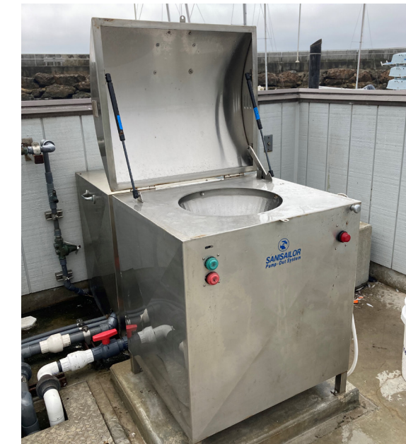
Motorized dump station Photo by TBF
