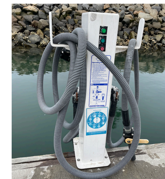
Pumpout unit retrofitted with a port-a-potty wand attachment Photo by TBF
