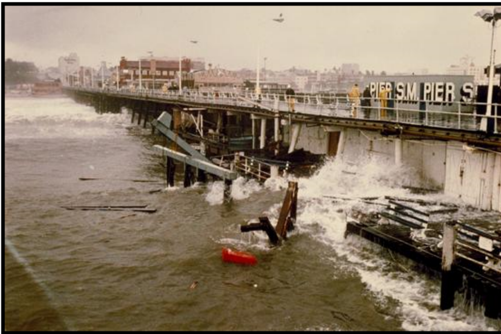
Figure 3. Breakwater protecting Santa Monica Pier (top; courtesy of Calisphere, October 24, 1936). The proposed project would enhance the poorly maintained breakwater to better protect Santa Monica Pier from storm damage, such as that from a 1983 storm (bottom; credit: Santa Monica Pier Collapse News Coverage, 1983 ).
